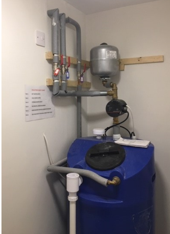
Cold Water Storage Tank and associated valves located in store
